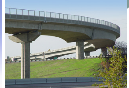
I-5: Beltline Flyover Bridge
