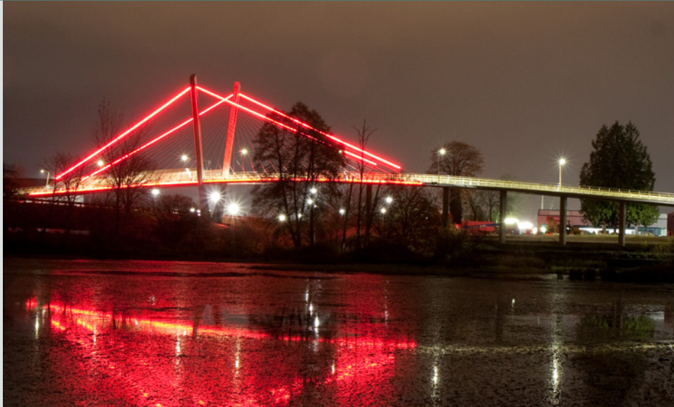
Delta Ponds Pedestrian Bridge
