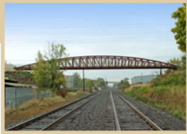
Pictured: Springwater Trail UPRR Pedestrian Bridge
