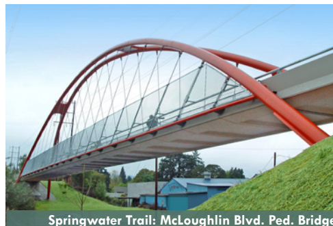
Springwater Trail: McLoughlin Blvd. Ped. Bridge
