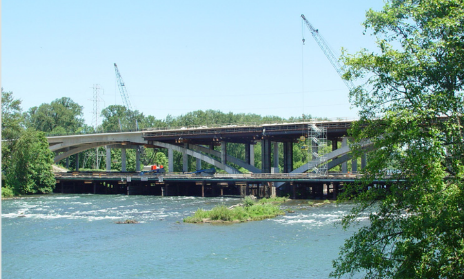
I-5 Willamette River Bridge
