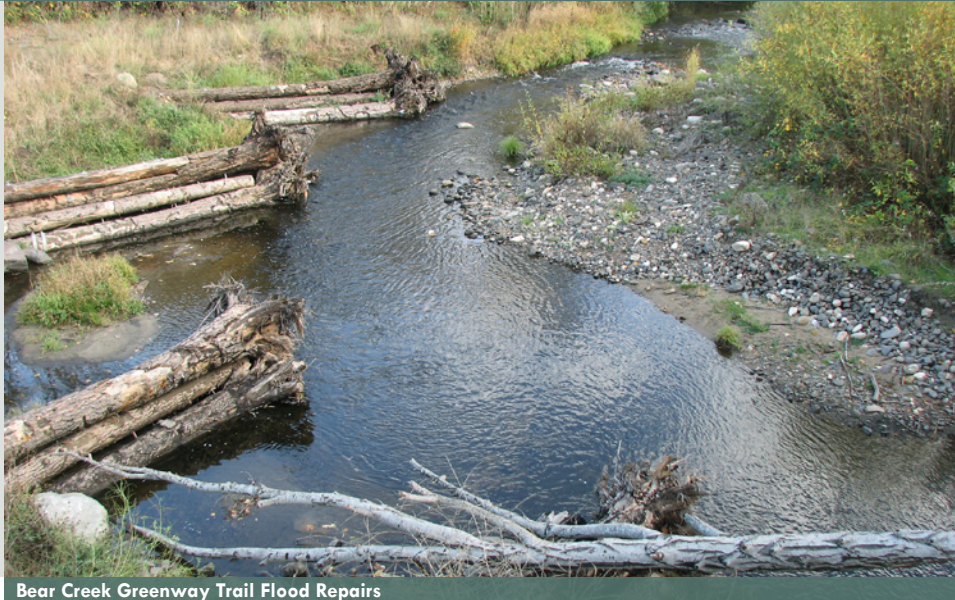
Bear Creek Greenway Trail Flood Repairs
