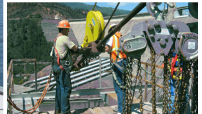
Shasta Dam Cableway Removal
