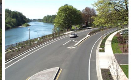
Ferry St. Bridge & Overpass Improvements
